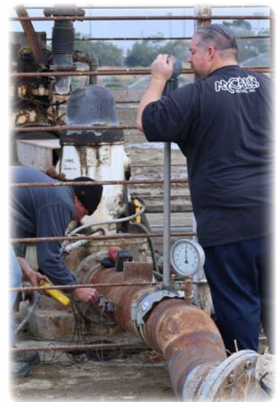
Testing Agricultural Meter for Accuracy
